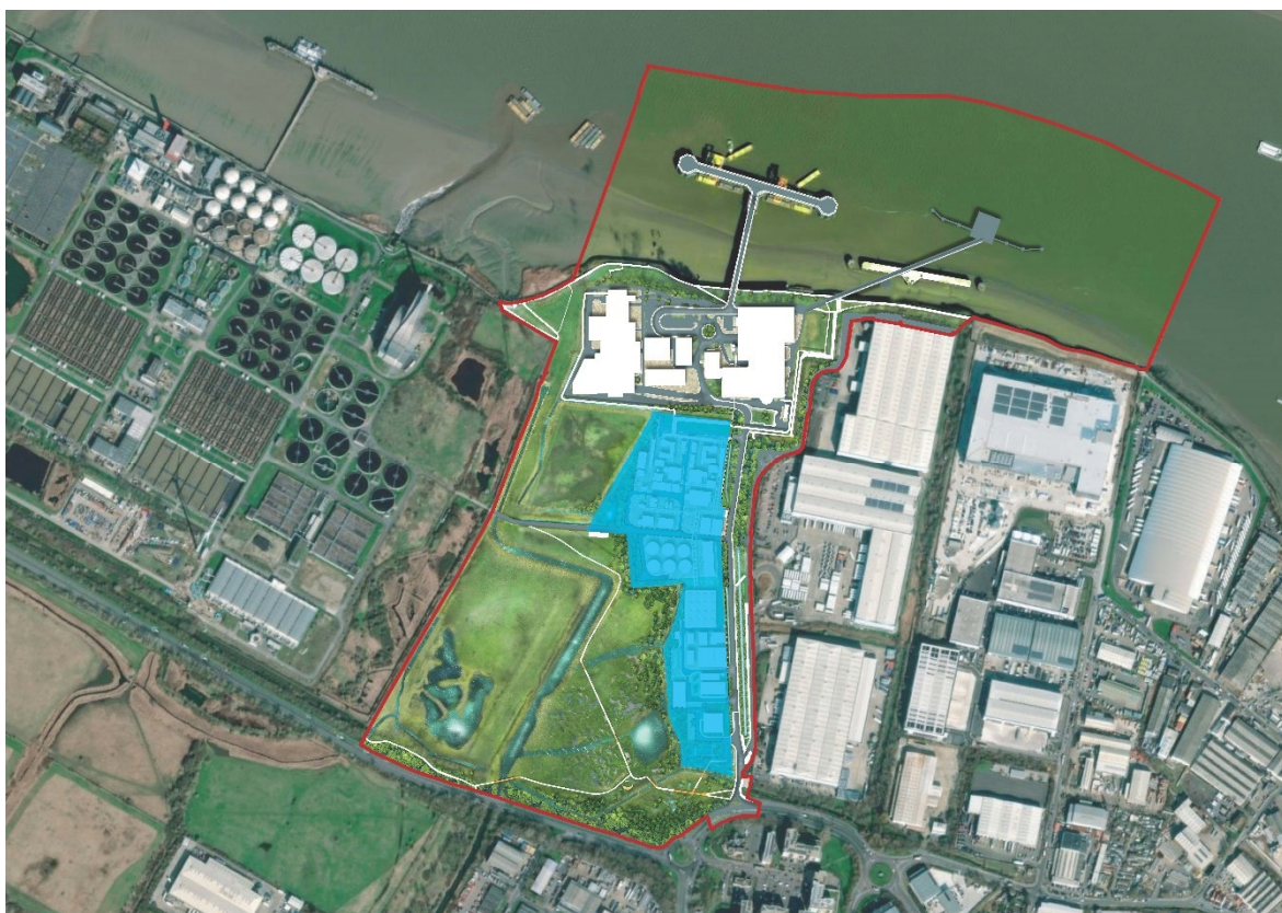
Figure 6 Carbon Capture Facility (CCF) Area
